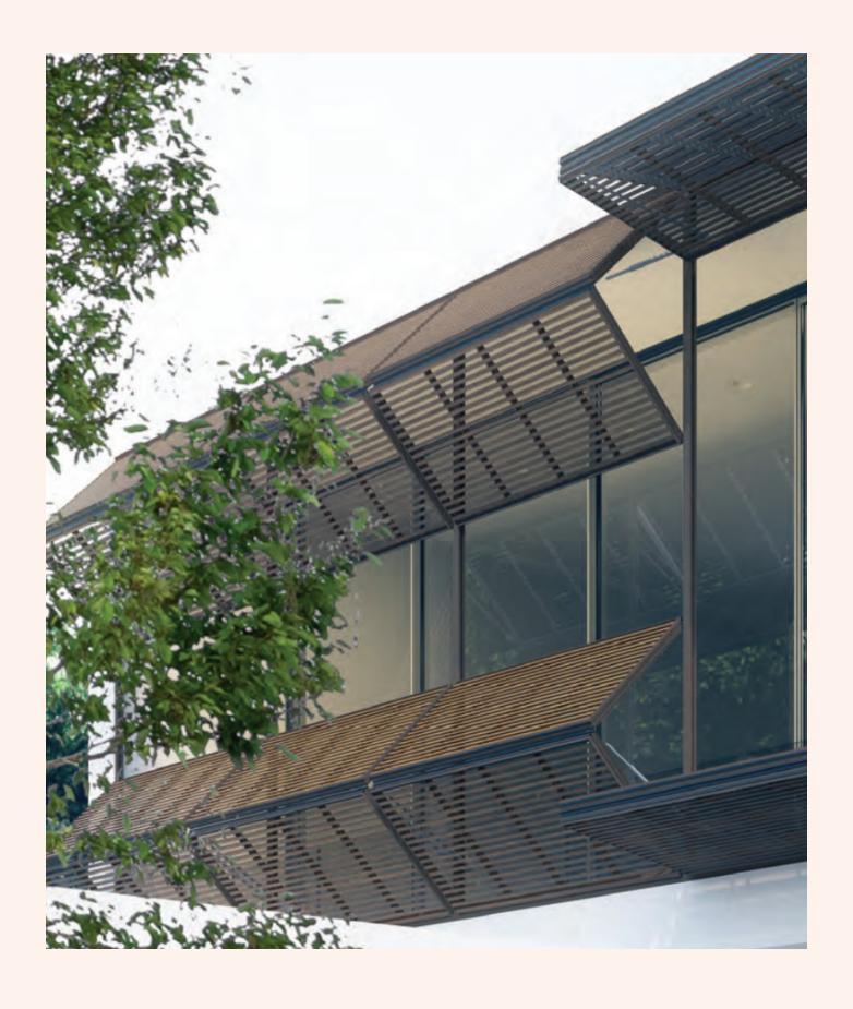
This new and innovative external facade shading system has been designed to allow for seamless integration with the external cladding of any building. Several cladding finishes are available to choose from to ensure this system meets specific design requirements.
